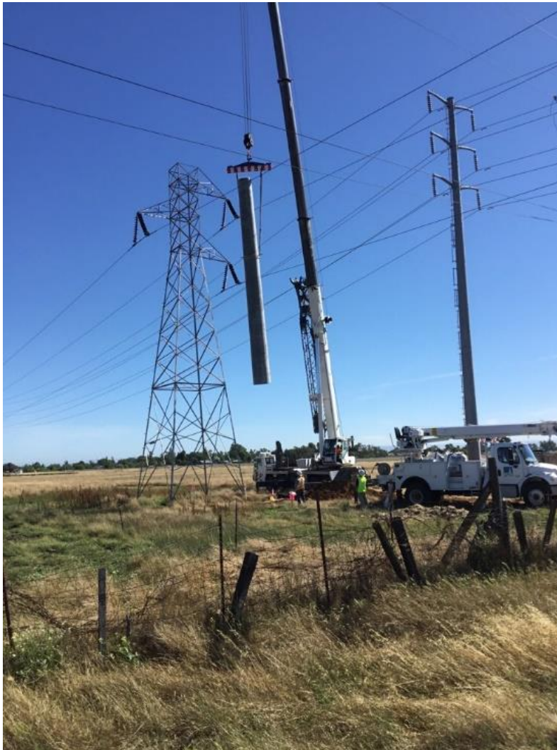
Photo 1: Crews placing an abutment at site 29/213.
