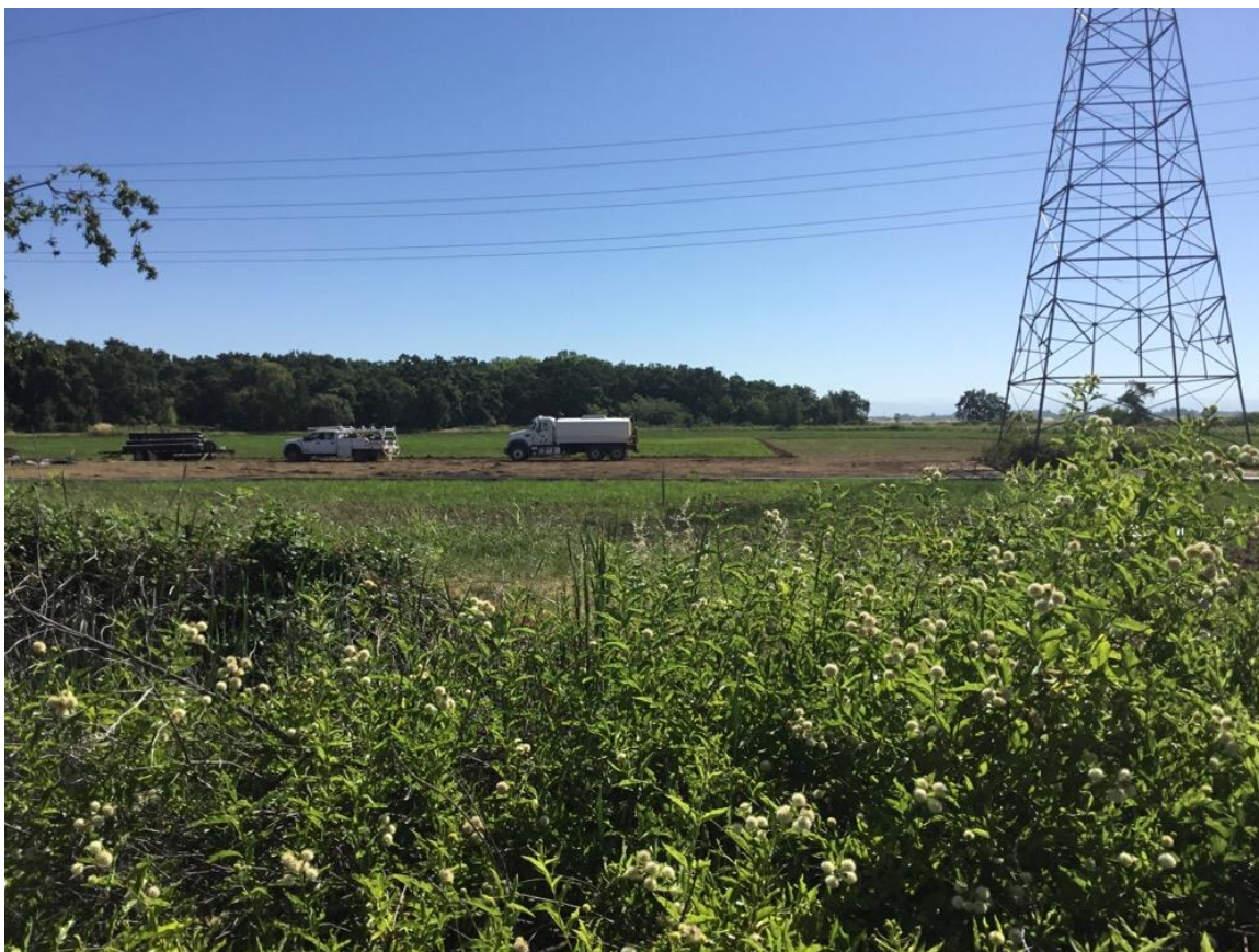
Photo 4: The CPUC EM observed a water truck at Pull Site (PS) 21/151 to suppress fugitive dust in accordance with APM AQ-2.
